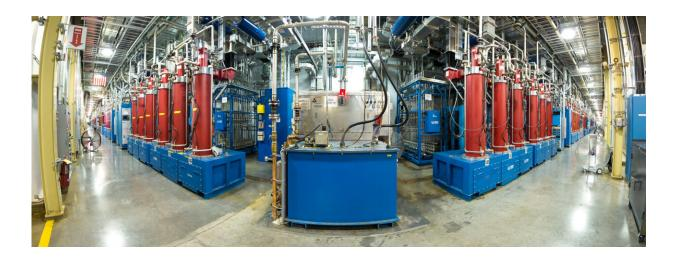
Upgrades to the particle accelerator enabling the record 1.7-megawatt beam power at the Spallation Neutron Source include adding 28 high-power radiofrequency klystrons (the red tubes) to provide higher power for the accelerator. Credit: Genevieve Martin/ORNL, U.S. Dept. of Energy
