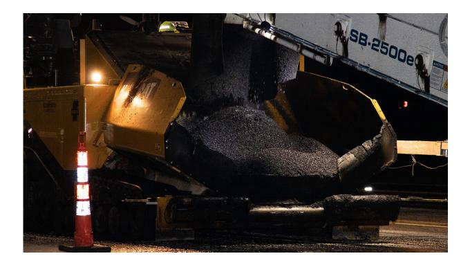
A pavement mixture using recycled plastic is applied to a section of Stadium Boulevard in Columbia near U.S. Highway 63 in 2021. Credit: University of Missouri
