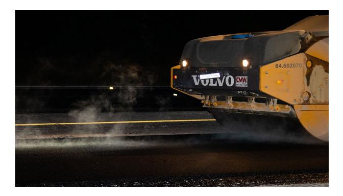
Steam rises from the newly poured plastic waste pavement mixture as an asphalt roller compacts the mixture into a smooth driving surface along Stadium Boulevard in Columbia in 2021. Credit: University of Missouri
