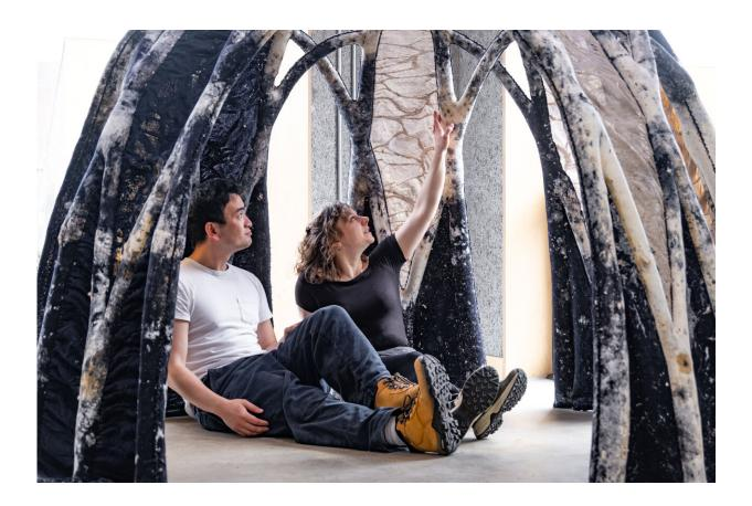
A 1.8m high, 2m diameter freestanding structure made of the BioKnit mycocrete using knitted formwork. Two people are sitting inside it. Credit: Hub for Biotechnology in the Built Environment.
