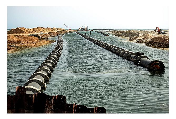
Pipes are laid to channel seawater to the Zarat Desalination Plant in Gabes in southeast Tunisia.
