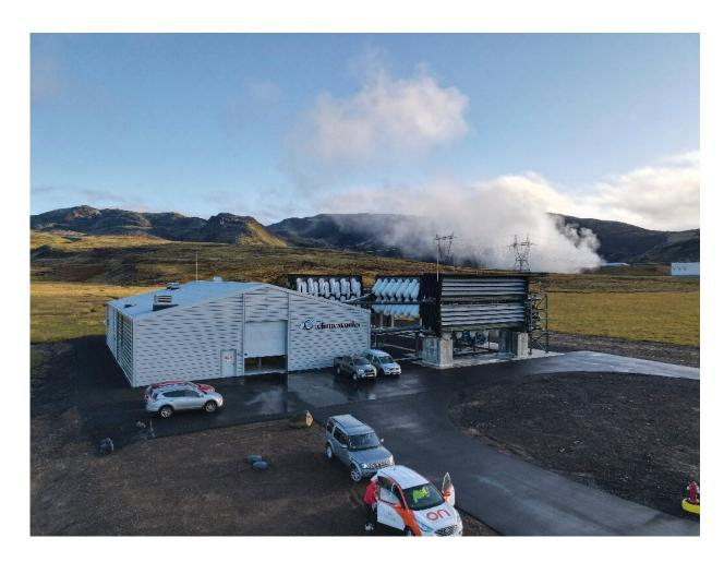
Climeworks "direct air capture" factory removes CO2 from the air.
