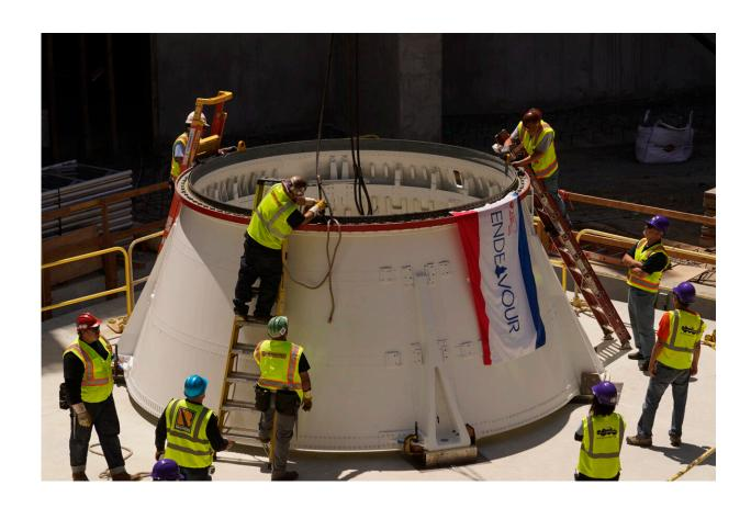
Technicians remove lifting lugs after placing the Space Shuttle Endeavour's Solid Rocket Aft Skirts on top of a seismic isolator pad in the Shuttle Gallery of at the Samuel Oschin Air and Space Center in Los Angeles, Thursday, July 20, 2023. The 20-story tall display which is currently under construction will stand atop an 1,800-ton concrete slab supported by so-called base isolators to protect Endeavour from earthquakes. Credit: AP Photo/Damian Dovarganes
