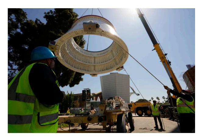
Workers used a crane to hoist the Solid Rocket Aft Skirts, the bottom segments of the boosters of the Space Shuttle Endeavour, before placing them on top of a seismic isolator pad inside the Shuttle Gallery at the Samuel Oschin Air and Space Center in Los Angeles, Thursday, July 20, 2023. Credit: AP Photo/Damian Dovarganes
