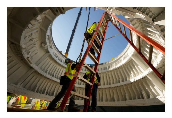
Technicians attach specialized lifting lugs to the top ring of the Solid Rocket Aft Skirts, the bottom segments of the boosters of the Space Shuttle Endeavour, before using a crane to place them on top of a seismic isolator pad inside the Shuttle Gallery at the Samuel Oschin Air and Space Center in Los Angeles, Thursday, July 20, 2023. Credit: AP Photo/Damian Dovarganes
