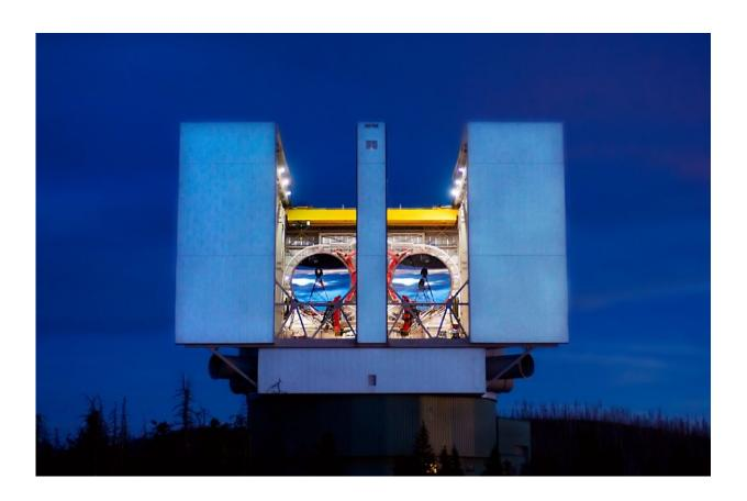
The Large Binocular Telescope in Arizona. The LBTI instrument combines infrared light from both 8.4m mirrors to image planets and disks around young and nearby stars. Credit: D. Steele, Large Binocular Telescope Observatory
