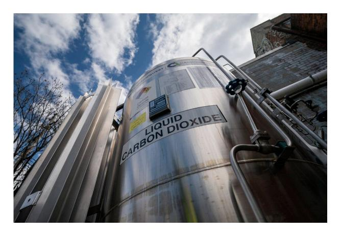
A liquid carbon dioxide containment unit stands outside the fabrication building of Glenwood Mason Supply Company, Tuesday, April 18, 2023, in the Brooklyn borough of New York. New York is forcing buildings to clean up, and several are experimenting with capturing carbon dioxide, cooling it into a liquid and mixing it into concrete where it turns into a mineral. Credit: AP Photo/John Minchillo
