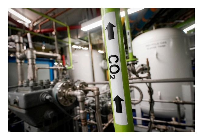
A liquid carbon dioxide pipe is labeled in a production room of The Grand Tier luxury apartment building, where the carbon byproduct of a natural gas fired water boiler is repurposed for industrial sale, Tuesday, April 18, 2023, in New York. New York is forcing buildings to clean up, and several are experimenting with capturing carbon dioxide, cooling it into a liquid and mixing it into concrete where it turns into a mineral. Credit: AP Photo/John Minchillo
