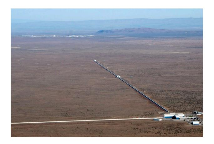
The LIGO detector in Hanford, Wash., uses lasers to measure the minuscule stretching of space caused by a gravitational wave. Credit: LIGO Laboratory
