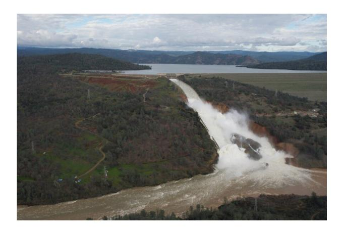
Water rapidly flows from the eroded Oroville Dam spillway in February 2017. The large gully to the right was caused by water cascading through a broken and damaged concrete surface. Credit: California Governor's Office of Emergency Services
