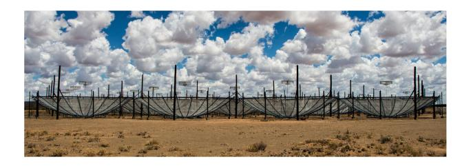
A view of HERA from 2017 January. The data in this work were taken during Phase I, when HERA was composed of 14 m parabolic dishes with sleeved dipole feeds in mesh cages suspended at prime focus. These feeds were later replaced with wide-band Vivaldi feeds, expanding HERA's bandwidth from 100–200 MHz (Phase I) to 50–250 MHz (Phase II). Credit: *The Astrophysical Journal* (2023). DOI: 10.3847/1538-4357/acaf50
