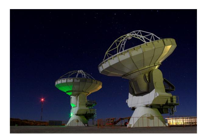
Two North American 12-meters sit under the stars at the ALMA Operations Support Facility (OSF). Towards the left of the image in the distance is the Holography Tower. The antennas are able to receive a signal from this tower and use it to make a map of their surfaces. The individual panels that make up their surface can then be adjusted so that the surface is as close to being perfect parabola as possible. Credit: Carlos Padilla
