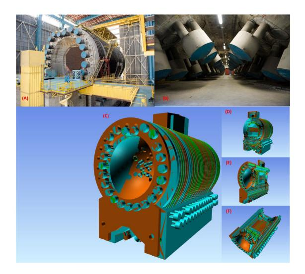
The G2 reactor. (A and B) Photographs from the North side and below the concrete cylinder, (C) CAD full view, and (D to F) cross sections along the three
