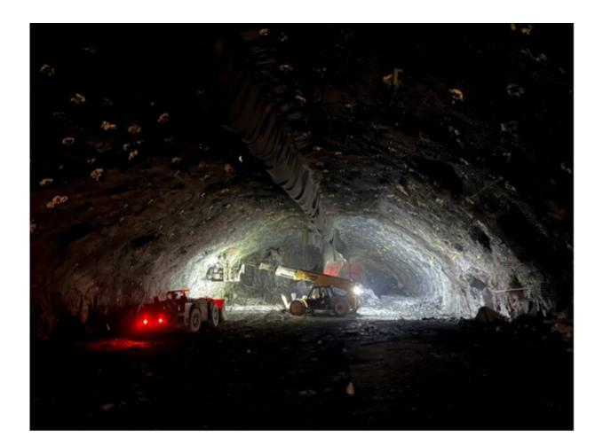
When complete later this year, this cavern will be around 500 feet long, 65 feet wide and 90 feet high. It will be one of three caverns that will provide space to house particle detector modules and other equipment for the Deep Underground Neutrino Experiment. Credit: David Smith, Fermilab
