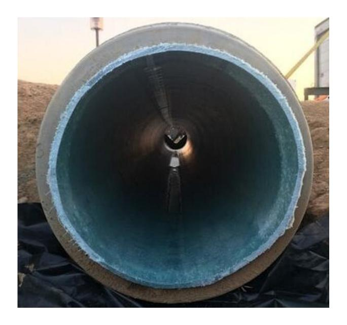
The blue cured-in-place pipe, or CIPP, can be seen inside this damaged storm sewer pipe. The CIPP was created by steam cooking the resin into the hard plastic. Credit: Andrew Whelton/Purdue University
