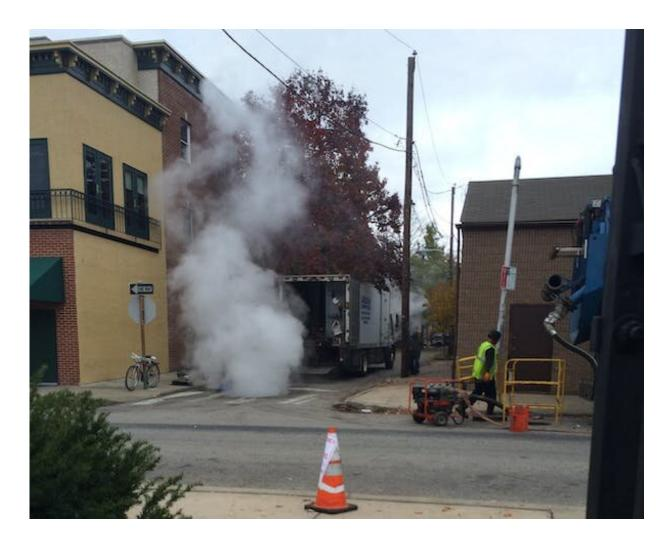
With this sewer pipe repair method, the chemical waste is blown into the air and can enter buildings through buried sewer pipes, plumbing, foundation cracks, windows, doors and HVAC units. Credit: <u>Andrew Whelton/Purdue University</u>
