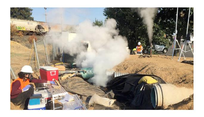
Purdue researchers perform testing during a CIPP installation in 2016. Credit: Purdue University
