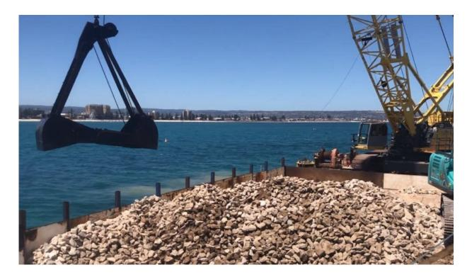
Restoring shellfish reefs starts with a limestone base, as in this construction image of the Glenelg oyster reef project. Credit: Maritime Constructions,  $\underline{CC}$ <u>BY</u>
