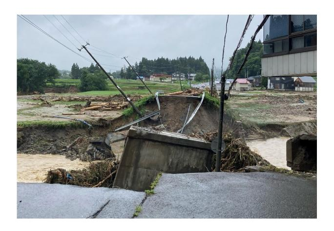
Omaki Bridge, which connects to the town of Iide, Yamagata Prefecture, collapsed after a river flooded.
