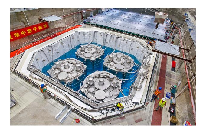
Bird's-eye view of the underground Daya Bay far detector hall during installation. The four antineutrino detectors are immersed in a large pool filled with ultra-pure water. Credit: Roy Kaltschmidt, Berkeley Lab
