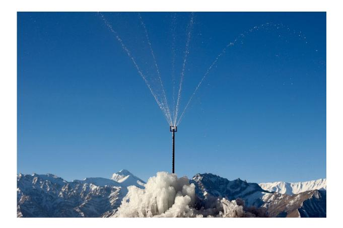
A fountain sprays water for an artificial ice reservoir in Ladakh, India. Low, steady flow over months can build ice towers 30 meters high. Meltwater from these structures irrigates crops in spring. Credit: Suryanarayanan Balasubramanian
