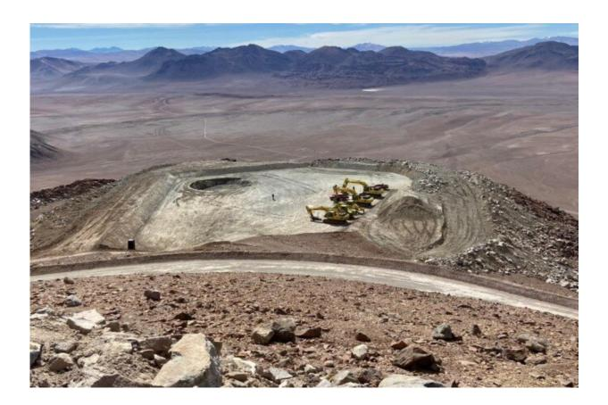
A hole 22 meters in diameter near the summit of Cerro Chajnantor in Chile's Atacama Desert, at an elevation of 18,400 feet stands ready for the cement foundation on which the Fred Young Submillimeter Telescope will one day rest. Credit: Cornell University
