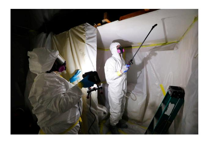
Asbestos Removal Technologies Inc., job superintendent Ryan Laitila, right, sprays amended water as job forman Megan Eberhart holds a light during asbestos abatement in Howell, Mich., Oct. 18, 2017. The Environmental Protection Agency on Tuesday, April 5, 2022, proposed a rule to finally ban asbestos, a carcinogen that is still used in some chlorine bleach, brake pads and other products and kills thousands of Americans every year. Credit: AP Photo/Paul Sancya, File
