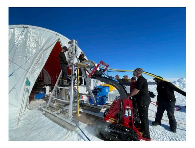
A group of engineers swarm around a frame to help lower equipment designed to melt a hole in the ice shelf. Credit: Craig Stevens/K862/NIWA, <u>CC BY-ND</u>
