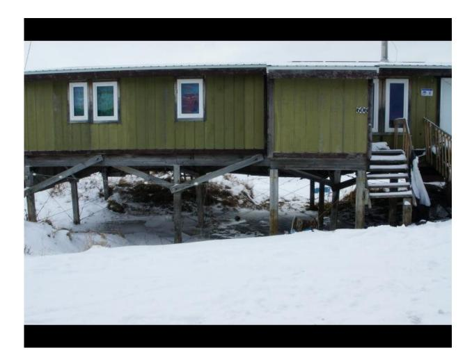
The amount of subsidence can be inferred by the distance from the bottom step to the ground in this photo of a building in Point Lay, Alaska. Credit: Bill Tracey
