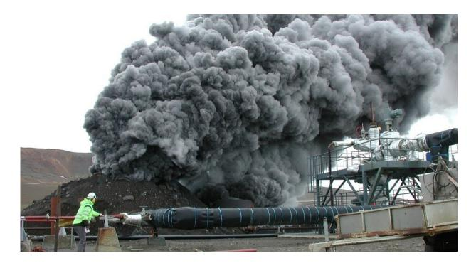
In 2009, a bore drill hit a pocket of 900 degree Celsius (1,650 Fahrenheit) magma by chance, at a depth of 2.1 kilometres.
