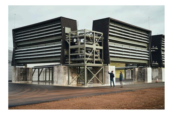
In this September 2021 image provided by Climeworks AG, CEOs Jan Wurzbacher and Christoph Gebald appear in front of an air-scrubbing machine where fans suck air into big, black collection boxes where the carbon dioxide accumulates on a filter at Climeworks' Orca plant near Reykjavik, Iceland. The Iceland plant is the largest such facility in the world, capturing about 4,000 metric tons of carbon dioxide per year. Credit: Climeworks AG via AP
