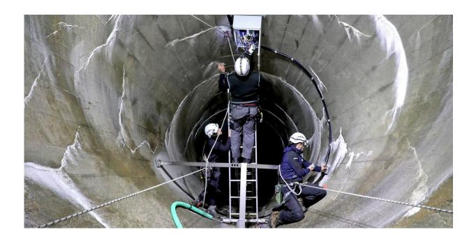
For the measurement campaigns, the research team first installed 16 custommade probes in the tunnel spillway of the 225 m high Luzzone Dam. Credit: VAW, D-BAUG / ETH Zurich
