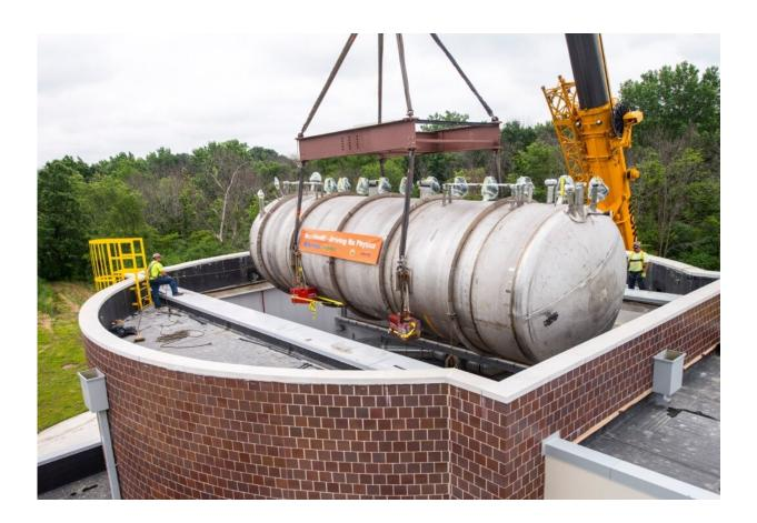
MicroBooNE detector being lowered into the experimental facility at Fermilab. Credit: Fermilab
