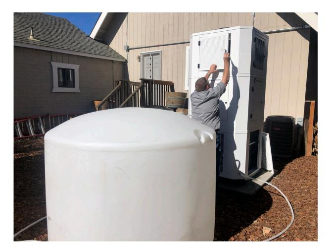
Ted Bowman, design engineer with Tsunami Products, installs a unit in homeowner Don Johnson's backyard in Benicia, Calif., Sept. 28, 2021. The recent invention can make water out of the air and in parched California, some homeowners are already buying the pricey devices. The air-to-water systems work like air conditioners by using coils to chill air, then collect water drops in a basin. Credit: AP Photo/Haven Daily
