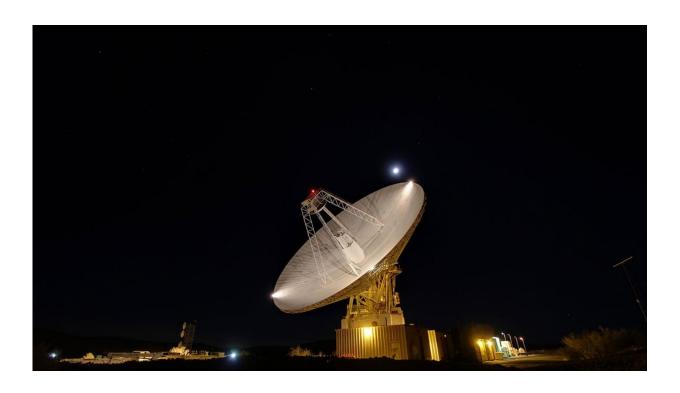
The 70-meter (330-foot) Deep Space Station 14 (DSS-14) is the largest Deep Space Network antenna at the Goldstone Deep Space Communications Complex near Barstow, California. Credit: NASA/JPL-Caltech
