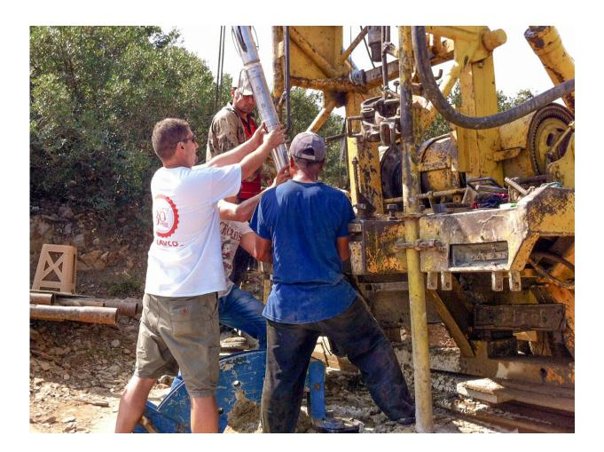
Installation of a strainmeter for a GONAF borehole in Turkey. Complementary to classical seismometers, these devices can also measure slow deformations in the subsurface down to the dimension of an atomic diameter  $(10^{-10} \text{ m})$ . Credit: Marco Bohnhoff, GFZ
