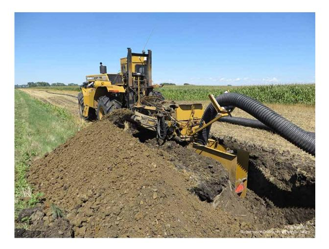
The installation of a drainage pipe. These drains help remove water from waterlogged fields, which helps crops grow better. Credit: J. Kjaersgaard
