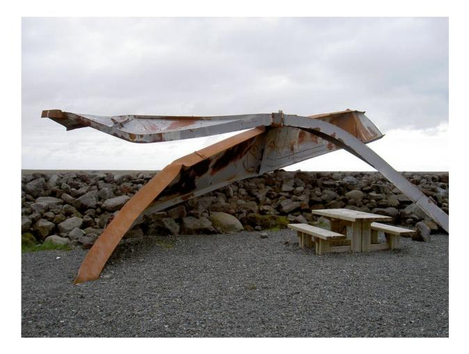
The twisted remains of a steel bridge destroyed by a glacial lake outburst flood in Iceland in 1996. Credit: (Chris 73/Wikimedia Commons), CC BY-SA
