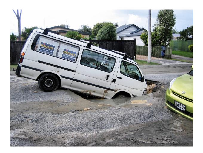
Sink holes and liquefaction on roads in Christchurch, New Zealand after 2011 earthquake. Credit: Martin Luff, CC BY-SA 2.0, via Wikimedia Commons
