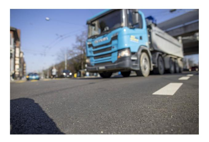
Load test: Since October 2020, rubber asphalt has been laid at a busy intersection in Zurich for test purposes. Credit: Gian Vaitl
