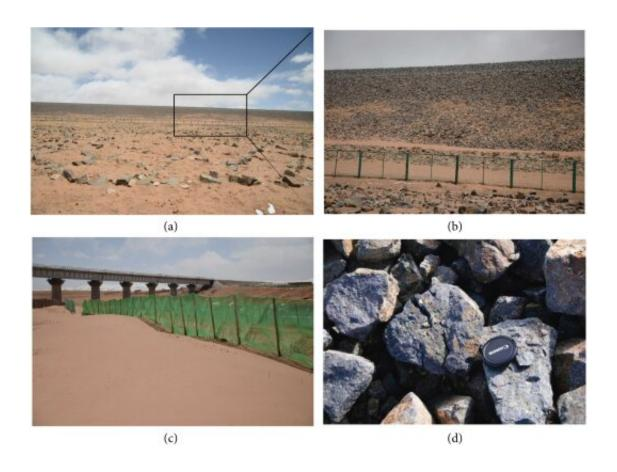
Wind-blown sand and rock-weathering of CRR embankment along the Qinghai-Tibet Railway. (a) Sand-filling of porous rock layer at the Honglianghe section; (b) close-view of sand-filling of the CRR; (c) prevalent sand prevention measure on the QTP; and (d) rock-weathering of the CRR caused by a severe environment. Credit: *Advances in Materials Science and Engineering* (2021). DOI: 10.1155/2021/5548638
