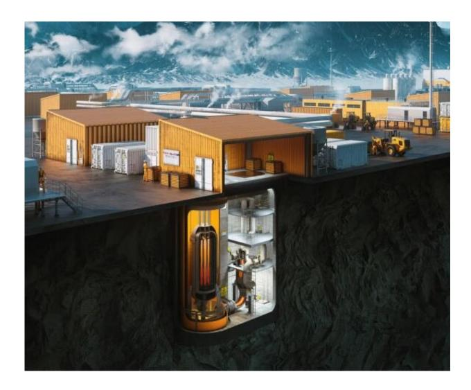
The Micro Modular Reactor (MMR<sup>TM</sup>) system is a fourth-generation nuclear energy system that delivers safe, clean, and cost-effective electricity and heat to remote mines, industry, and communities. It is the leading SMR project in Canada and the first so called "fission battery" concept worldwide. Credit: USNC
