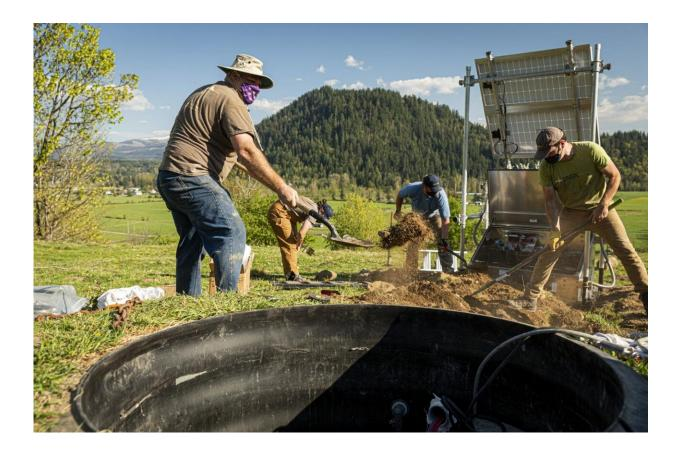
A team from the UW-based Pacific Northwest Seismic Network installs a new solar panel array at a seismic monitoring site in Enumclaw, Washington, on April 20, 2021. The seismometer, one of hundreds that provide data for ShakeAlert, is in the hole in the foreground. A trench brings cables to the newly installed solar panels, on the right, that power the system, and an aluminum box containing electronics that digitize and transmit the seismic data. Credit: Mark
