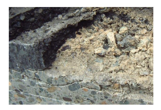
A close-up of a bridge, showing deteriorated asphalt pavement and concrete. Credit: Akihiro Moriyoshi
