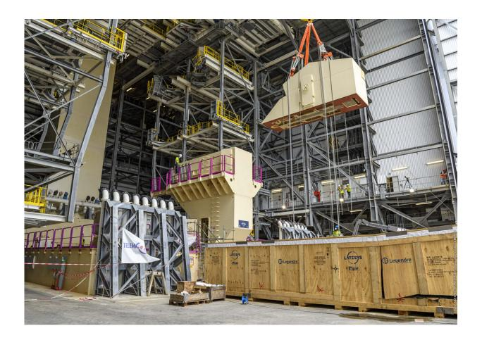
One of the mini-masts is installed on the Ariane 6 launch pad in preparation for combined tests with the cryogenic systems that will supply liquid oxygen and liquid hydrogen to the launch vehicle. Credit: ESA/CNES/Arianespace
