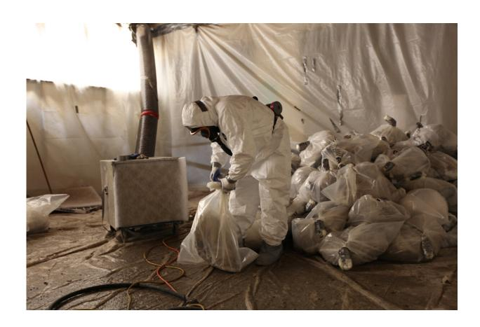
Friable asbestos ceiling materials are removed and double bagged at a quarantined facility at Naval Base Coronado Naval Air Station North Island. Credit: Jimmy Johnson/U.S. Navy
