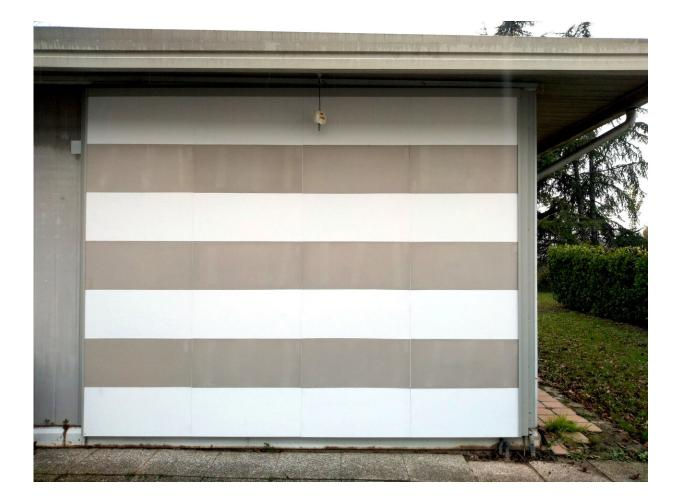
Panels made from recycled concrete can provide thermal insulation for buildings. Credit: Matteo Panizza / Sergio Tamburini
