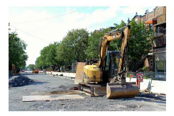
Construction work near trees often involves excavation that damages part of the root system. Work is carried out here on St-Denis Street in Montréal. Author provided
