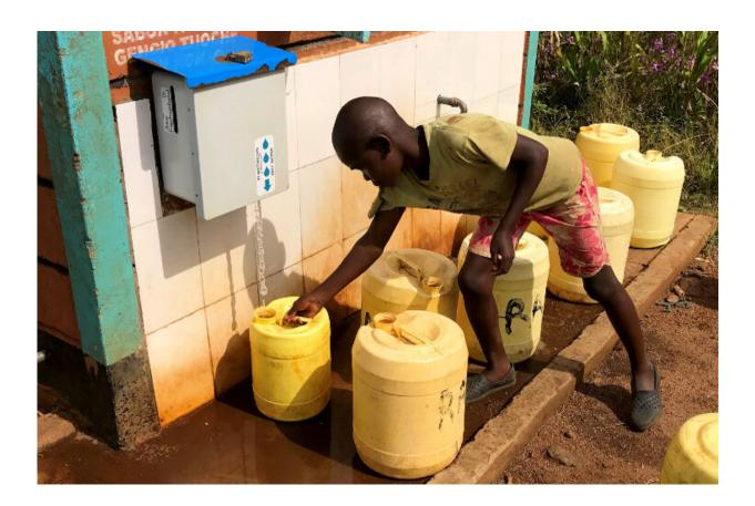
The chlorine treatment device requires little maintenance and no change in collection of water from the tap. Credit: Amy Pickering
