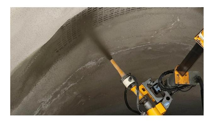
The use of shotcrete is one of the most important support measures in tunnel construction. Credit: ASSpC - TU Graz
