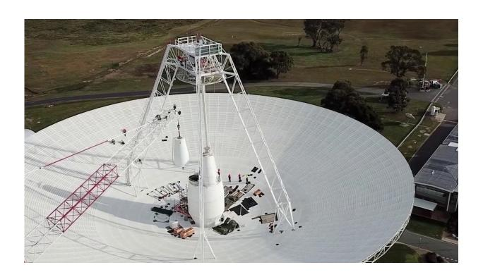
Crews conduct critical upgrades and repairs to the 70-meter-wide (230-foot-wide) radio antenna Deep Space Station 43 in Canberra, Australia. In this clip, one of the antenna's white feed cones (which house portions of the antenna receivers) is being moved by a crane. Credit: CSIRO
