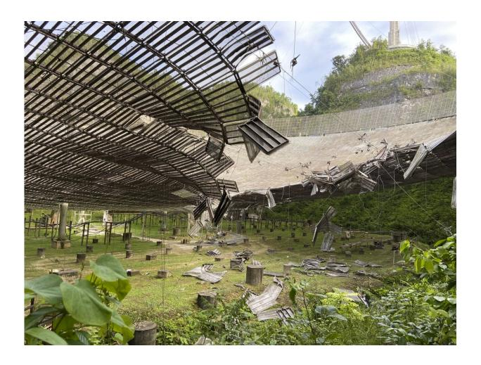
In this Tuesday, Aug. 11, 2020 file photo, provided by the Arecibo Observatory, shows the damage done by a broken cable that supported a metal platform, creating a 100-foot (30-meter) gash to the radio telescope's reflector dish in Arecibo, Puerto Rico. Giant, aging cables that support the radio telescopes are slowly unraveling in this U.S. territory, threatening scientific projects that researchers say can't be done elsewhere on the planet. (Arecibo Observatory via
