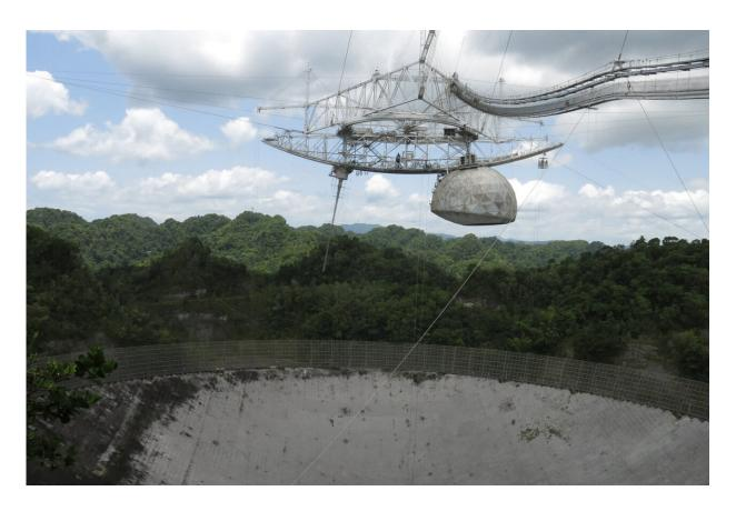
This July 13, 2016 file photo shows one of the largest single-dish radio telescopes at the Arecibo Observatory in Arecibo, Puerto Rico. Giant, aging cables that support the radio telescopes are slowly unraveling in this U.S. territory, threatening scientific projects that researchers say can't be done elsewhere on the planet. (AP Photo/Danica Coto, File)
