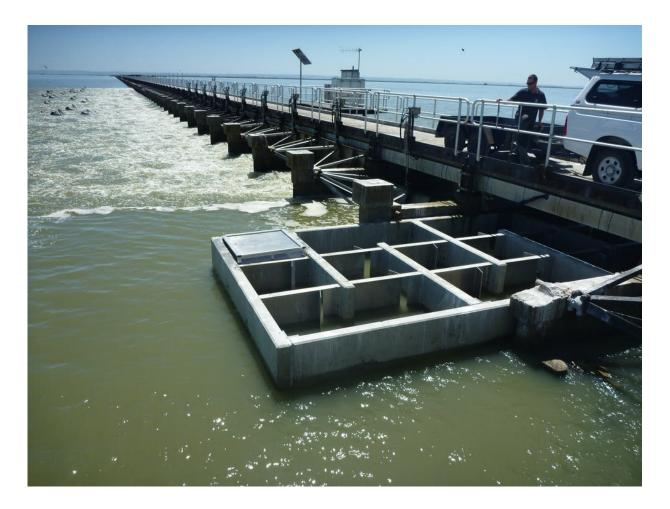
A fish ladder on the Murray Barrages. Fish swim through this structure to move from the estuary.into the freshwater lakes and River Murray. Without fish ladders, fish are seldom able to move past the barrages. Credit: Brenton Zampatti, Author provided
