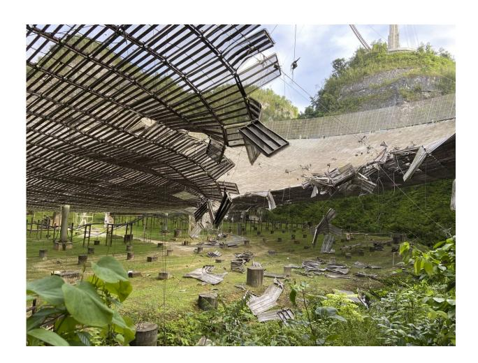
In this Tuesday, Aug. 11, 2020 file photo, provided by the Arecibo Observatory, shows the damage done by a broken cable that supported a metal platform, creating a 100-foot (30-meter) gash to the radio telescope's reflector dish in Arecibo, Puerto Rico. Giant, aging cables that support the radio telescopes are slowly unraveling in this U.S. territory, threatening scientific projects that researchers say can't be done elsewhere on the planet. (Arecibo Observatory via
