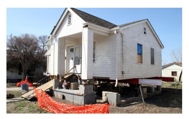
New Orleans, LA, March 8, 2006 - This house in Gentilly is in the process of being elevated above the base flood elevation adopted by the community in result of flooding from Hurricane Katrina. The homeowner will raise the house a total of 11' and has received the Increased Cost of Compliance (ICC) benefit included with his National Flood Insurance Program (NFIP) policy because of his compliance to the community's floodplain management ordinance. Credit: Robert Kaufmann/FEMA
